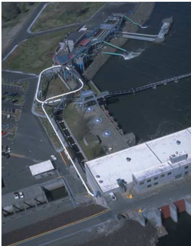
Figure 6. Smolt processing facility at the McNary Dam on the Columbia River (left) reroutes young fish migrating to sea, either by sending them through a network of tunnels back into the river but away from the deadly turbines, or by directing the fish into trucks or barges (below) that transport them past the McNary and three other downstream dams. Not all populations of salmon benefit equally from systems like this one, however: In a recent study, 95 percent of stream-type chinook were successfully guided away from the turbines at McNary Dam, whereas only 62 percent of ocean-type chinook were diverted. (Courtesy of PIT Tag Program, Pacific States Marine Fisheries Commission.)
