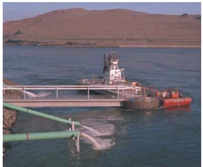
Figure 6. Smolt processing facility at the McNary Dam on the Columbia River (left) reroutes young fish migrating to sea, either by sending them through a network of tunnels back into the river but away from the deadly turbines, or by directing the fish into trucks or barges (below) that transport them past the McNary and three other downstream dams. Not all populations of salmon benefit equally from systems like this one, however: In a recent study, 95 percent of stream-type chinook were successfully guided away from the turbines at McNary Dam, whereas only 62 percent of ocean-type chinook were diverted. (Courtesy of PIT Tag Program, Pacific States Marine Fisheries Commission.)
