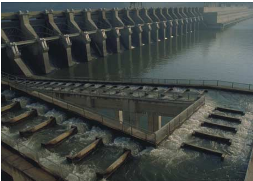
Figure 5. Fish ladders (such as this one at the John Day Dam near Rufus, Oregon, 216 miles from the mouth of the Columbia River) have been built to assist salmon migrating to their spawning grounds. Fish ladders resemble a series of small waterfalls; salmon swim or jump from one step to the next until they reach the top of the dam. The introduction of fish ladders at certain dams has improved the survival rates for salmon migrating upstream. Nevertheless, the presence of dams has transformed the environment in which the fish migrate, converting swiftly flowing rivers into series of slow-moving reservoirs punctuated by dams. (Courtesy of the U.S. Army Corps of Engineers.)
